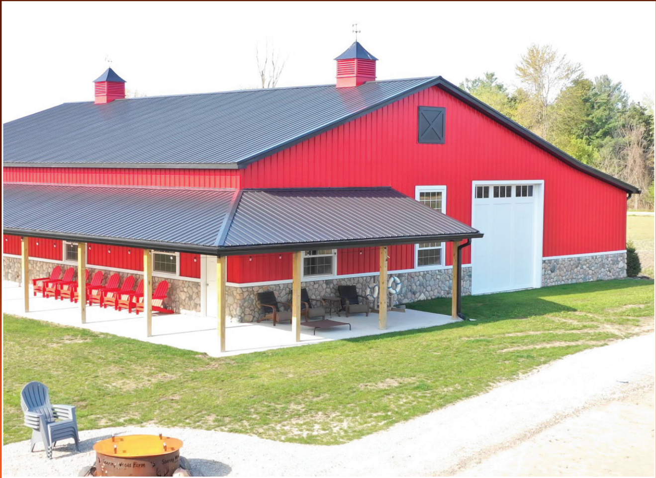
PHOTO COURTESY: ORCHARD CONSTRUCTION
