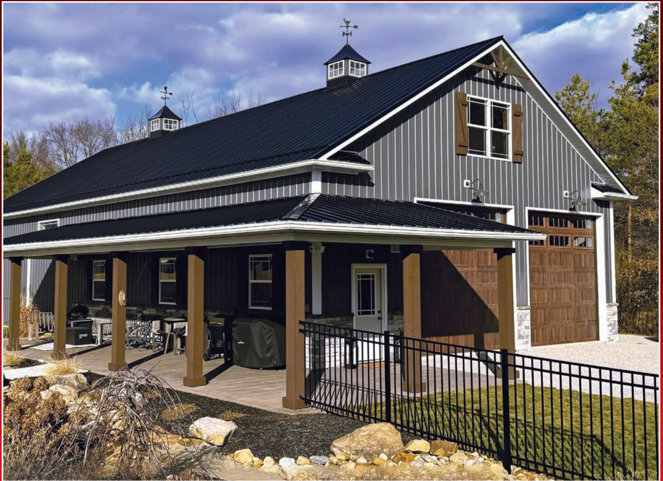
PHOTO COURTESY: POLE BARN'S DIRECT
