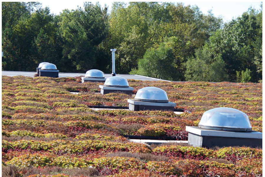
Solatube natural lighting tubes incorporated into a living roof system. PHOTO COURTESY OF KINGSPAN LIGHT + AIR NORTH AMERICA
