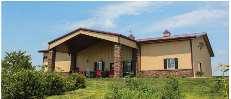
Shown during and after construction is this hybrid-built toy shed used by its owners as a garage, gym and workshop in Maryville, Missouri. Perka Building photo.
