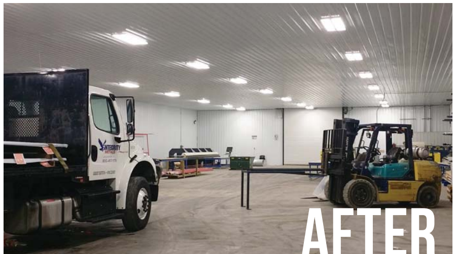
Integrity is now back to full production after months of rebuilding. Integrity photo
