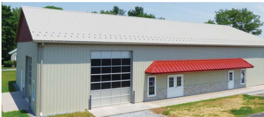
Products from Levi's were used from start to finish in the construction process of this new pole barn, ones you can't even see. Levi's is one source for all metal building fasteners, snow guard and accessory needs.
