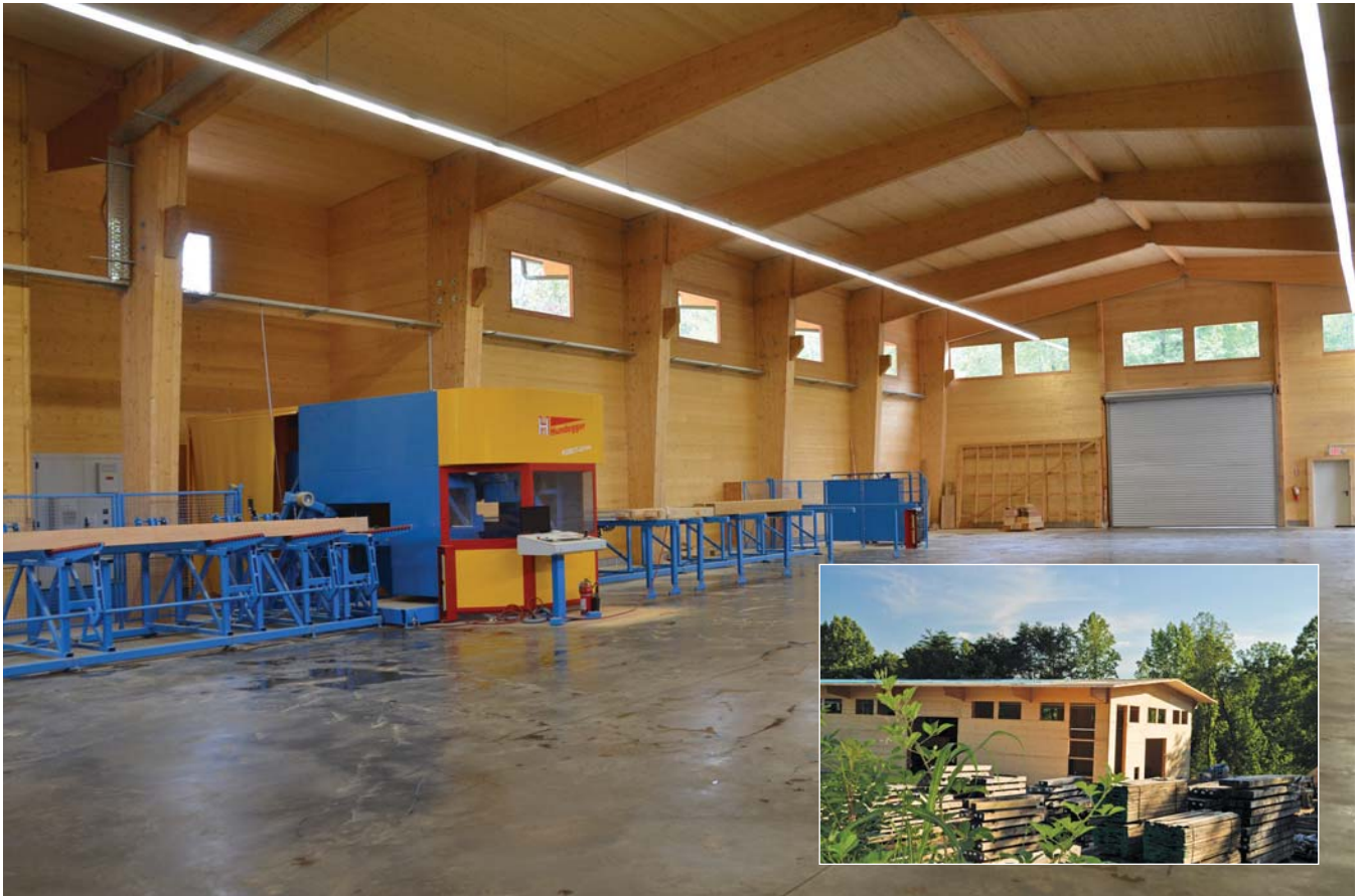
Sauter's new CLT building houses a new Hundegger jointery machine he can use for his existing timber-frame business as well as cross-laminated timber. Sauter photos
