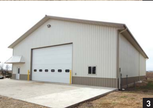
1. The SIP shop and storage shed with 8-inch walls (left), and a SIP storage shed. 2. The 48 x 68 SIP shop and storage shed. 3. The 60 x 88 SIP shop. 4. The 74 x 152 post-frame storage shed. 5. This interior view of the upper loft in the 48 x 68 foot SIP shop and storage shed shows the 24 x 68 foot recreation room. Photo credit: EPS Buildings
