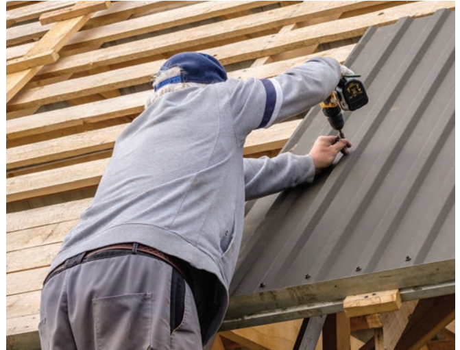
Metal-to-wood fastening. COURTESY OF TRIANGLE FASTENER CORPORATION
