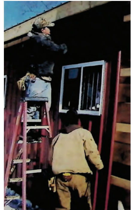
Brescia Buildings crew members hang the siding for the barn in February. The barn would have been finished earlier in 2000, but winter storms held up construction.
