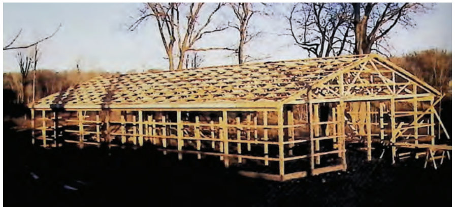
After holes for the columns were drilled in December, framing for the 36-ft. x 72-ft., 10-stall horse barn was finished, thanks to lumber donations from many Connecticut lumber companies and Brescia Buildings.
