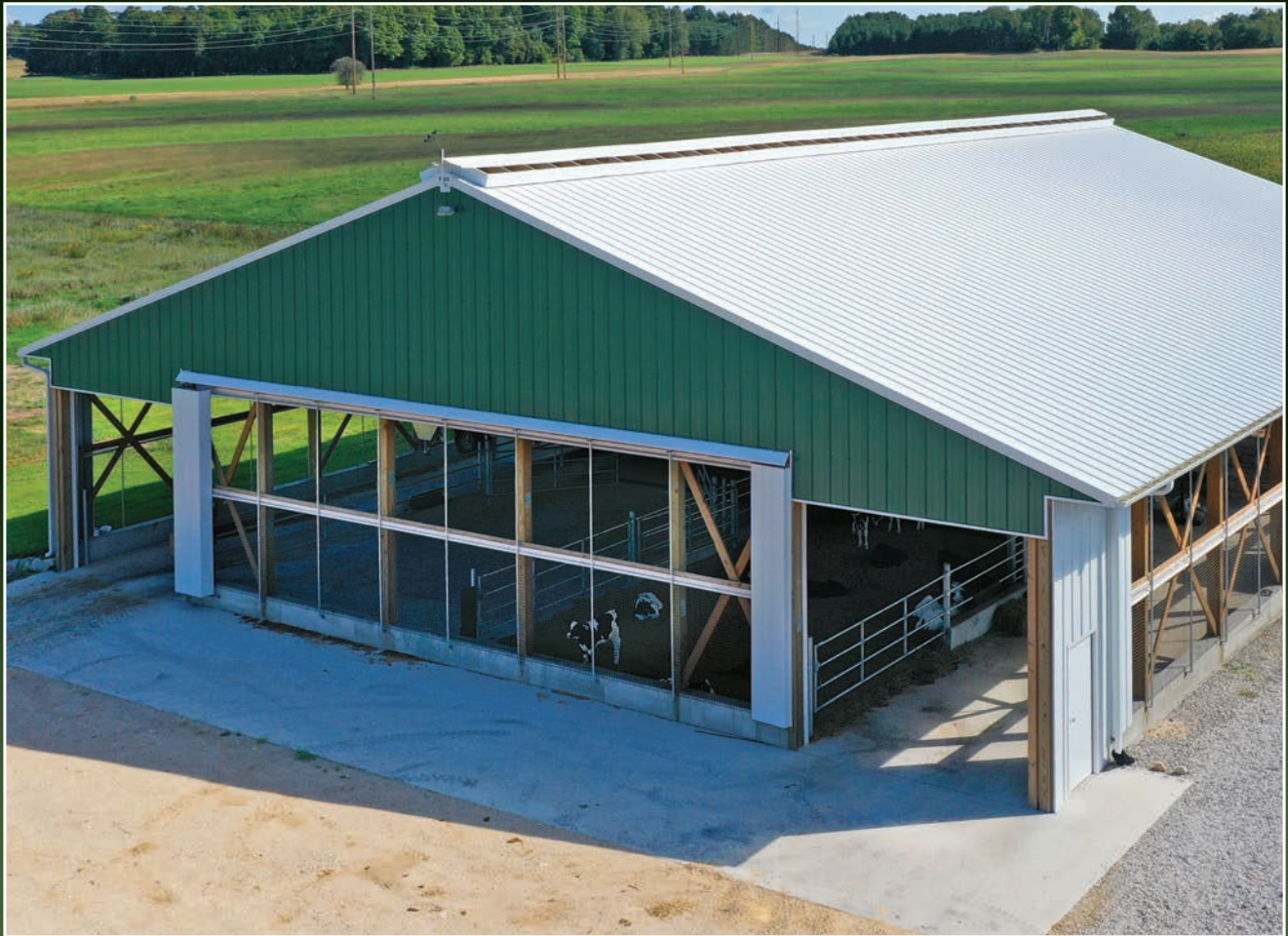
PHOTO COURTESY: WICK BUILDINGS
