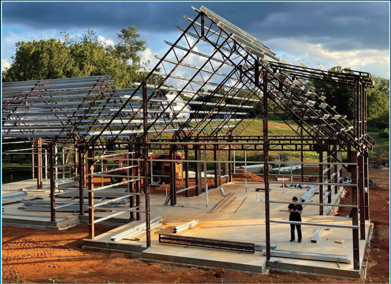
PHOTO COURTESY: WORLDWIDE STEEL BUILDINGS
