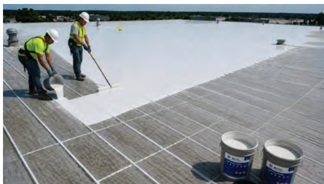
Figure 3. Detailing the penetrations. The crew applies the product using medium-nap rollers meant for solvent-based products.
