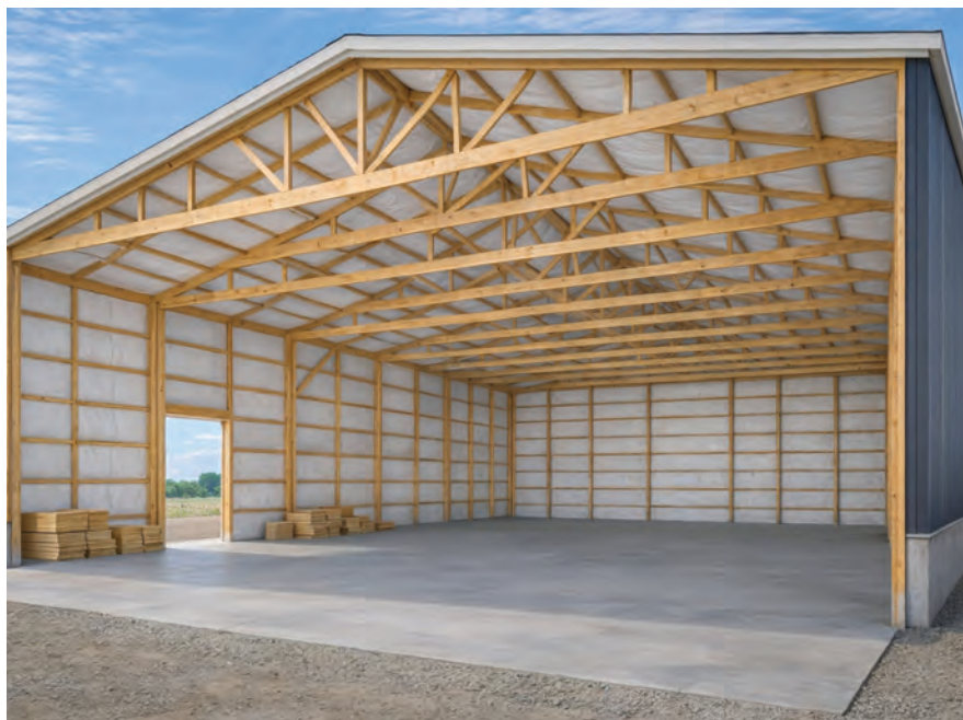
Applying insulation and metal together gives the installer a stable working surface and protects the insulation from wind and jobsite damage.
