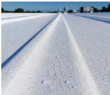
Figure 4. After, up close. Another significant benefit is that it waterproofs within 3 hours of application.
