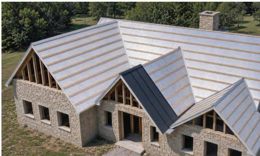
Furring strips below metal panels help accommodate expansion and contraction.
