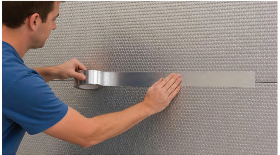
Seal every seam for best performance. PHOTOS COURTESY OF RFOIL
