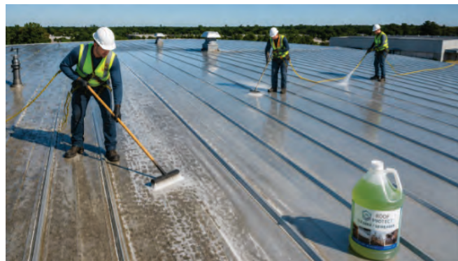
Figure 2. Applying Roof Protect. Crew scrubbing and rinsing from bottom to top before any coating goes down.
